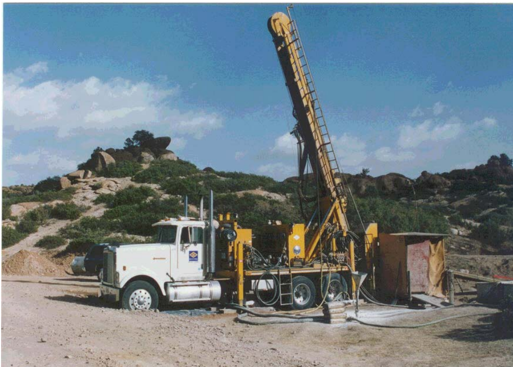
Figure 1 CS 4000 Core Drill Rig
